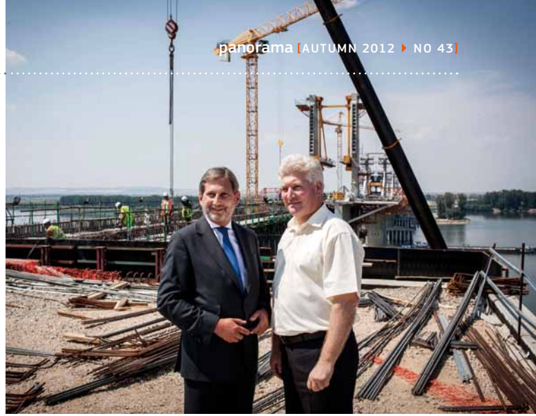
The Vidin-Calafat bridge between Bulgaria and Romania, progressing towards completion at the end of 2012, and part of the trans-European transport network which will aid connections between north west Bulgaria, south west Romania and eastern Hungary.
