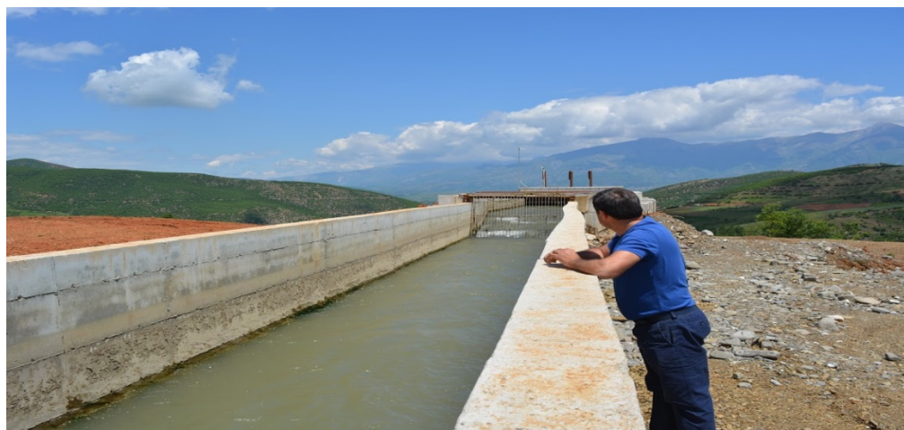
Small Hydropower Plant in Librazhd, Albania.
