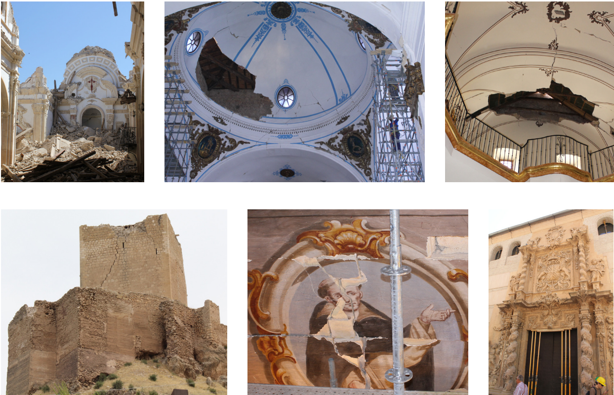
Figure 5. Examples of heritage assets damaged by the Lorca 2011 earthquake. Source: Photos courtesy of Xavier Romão and Esmeralda Paupério.
