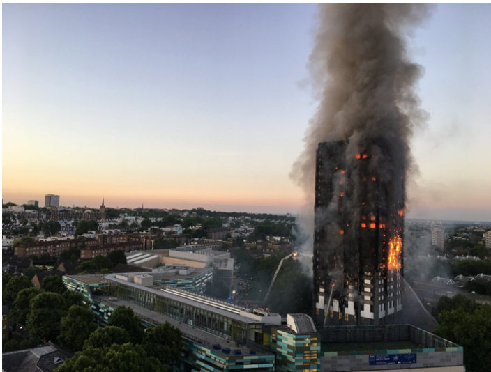
Figure 1. Grenfell Tower block, 4.00, 15 June 2017 Source: Natalie_Oxford, 2017
