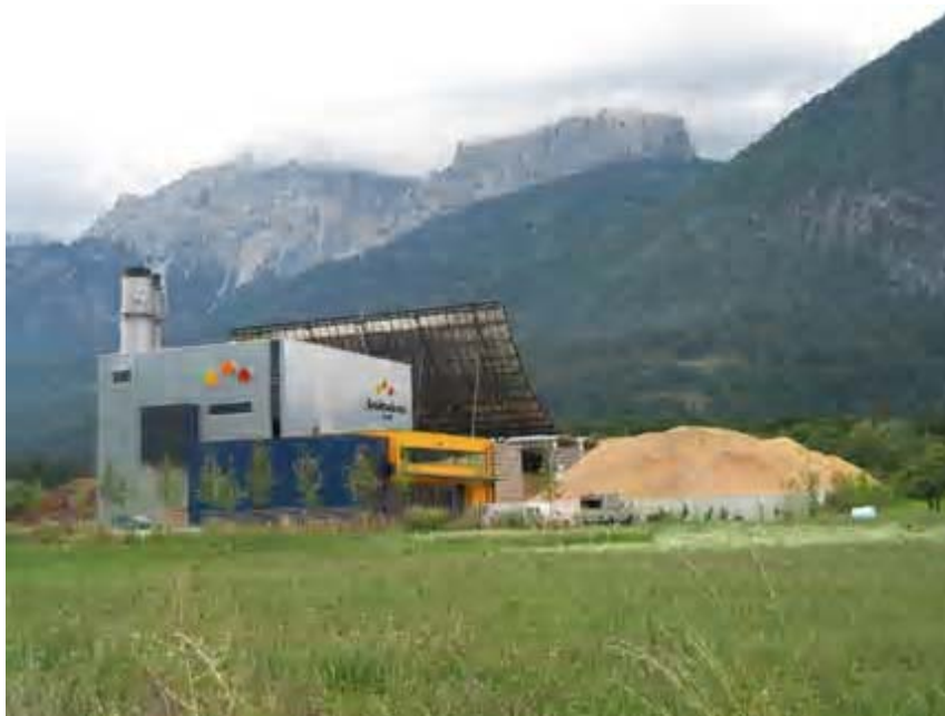
Figure 3.1: Biomass fired ORC co-generative district heating plant in Lienz, Austria /1/
