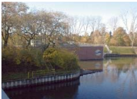
Figure 4: Herrenhausen Mini-Hydro Plant
