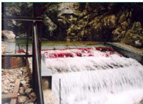
Figure 5: Small Hydro Plant at Anatoliki
