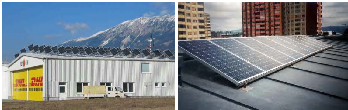
Figure 3.4: First 1,1 kW PV plant in Ljubljana and the latest biggest 16,3 kW PV plant in Airport Bled
