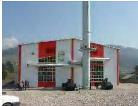
Figure 4.4: The thermal plant at Vatra Dornei.
