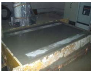
Figure 9. Founding of generator
