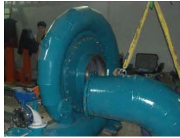
Figure 11. Francis turbine - installation
