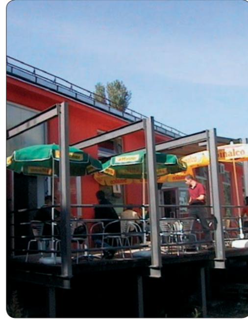
ACCESS center after renovation
