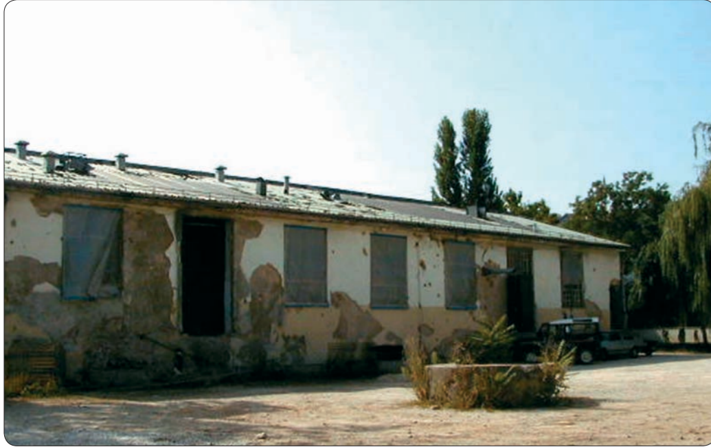
Location of the future ACCESS center before renovation
