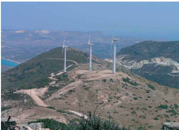
2,9 MW wind park on Milos Island
