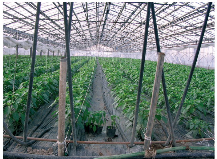
Geothermally heated greenhouse in Bansko (Podbelasica region)
