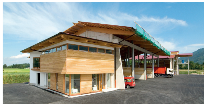
Biomass Centre Achental
