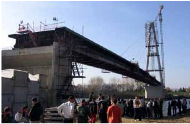
Bridge over the river Tisa in Ada – students' excursion
