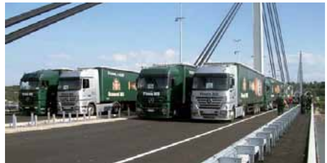
Trial load on the bridge Sloboda – Novi Sad
